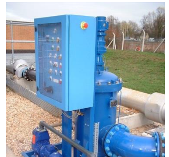
ABOVE: BOLLFILTER Automatic Type 6.18 installation at Thames Water's Grimsbury Water Treatment plant for protection of Ion Removal System.
