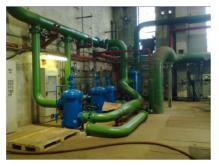
Fig. 2: Installation of BOLLFILTER system with pre-filter (background)
