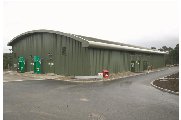
TOP. Dissolved Air Flotation plant at Lound.
