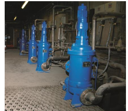
TOP. Images from the SMACC Continuous Casting Line. CENTRE. Kevin Davis, Outokumpu Engineer. BOTTOM. Part of the Installation of BOLLFILTER Automatic Type 6.18 serving the central cooling water system.
