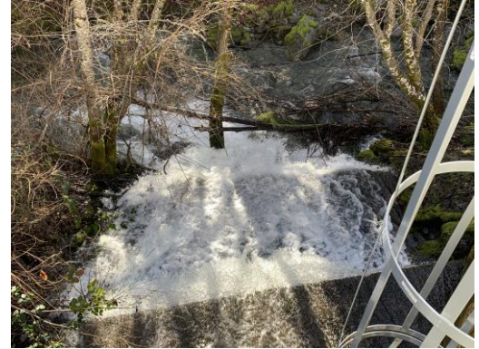
Water Source for Bearing Seal Water
