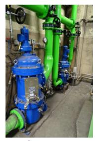
aquaBoll® automatic filter in the cooling process
