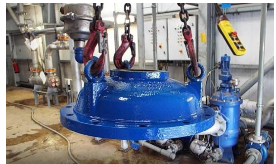
BOLLFILTER Engineer carefully repairing rust damage
